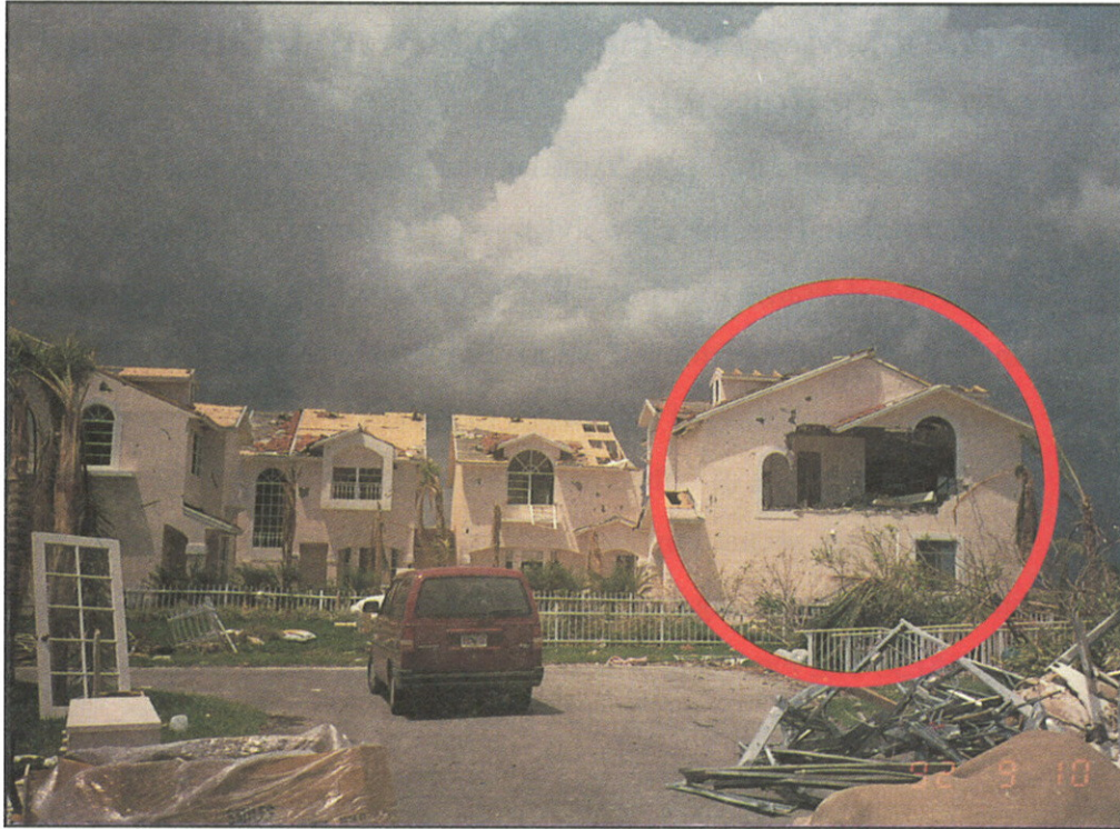
FIGURE 16. Two-story masonry buildings. Lack of continuous tie-beam led to failure of wall that was already weakened in design by window openings.
