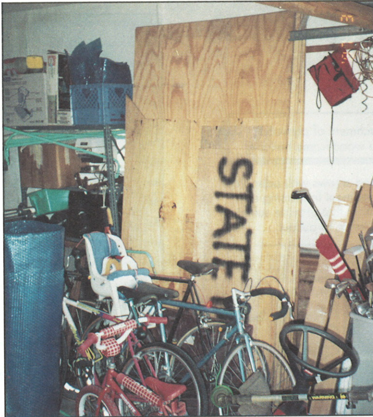
FIGURE 50. Previously purchased plywood stored for use as openings protection during storm conditions.
