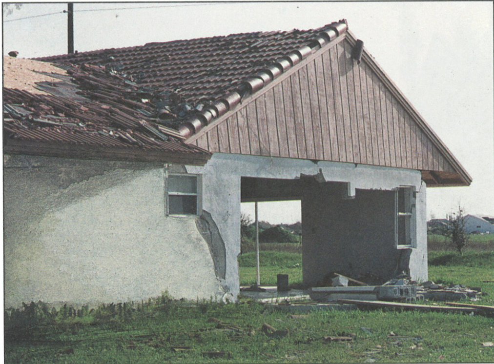
FIGURE 15. Masonry construction building. Wall separated from building envelope due to inadequate vertical wall reinforcing in connection to horizontal tie-beam.
