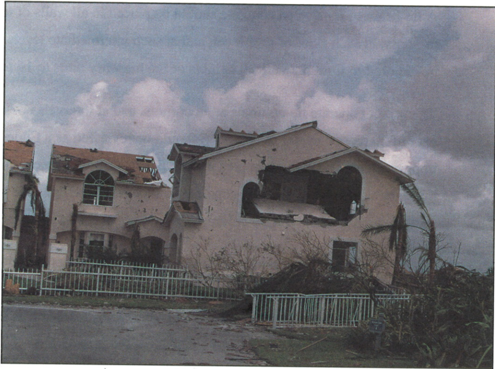
FIGURE 65. End wall failure. Freestanding concrete masonry wall has discontinuous tie-beam.
